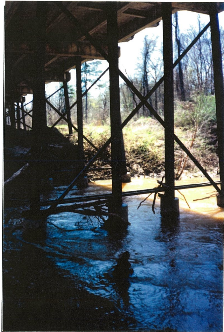
Figure 8. --Bents 11 and 12 of structure 124021500200 on Route SC 215, crossing the Sandy River in Chester County, South Carolina, showing the 2.5-ft diameter, concrete collars at the pile bases (April 20, 1993).
